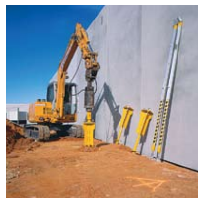
2. Install each brace anchor where marked anytime before erection of the precast concrete panels.
