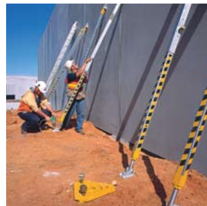
3. Attach the foot of the brace to the brace anchor and fix the head of the brace to the precast concrete panel.
